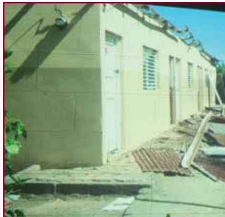
The school before construction began.
